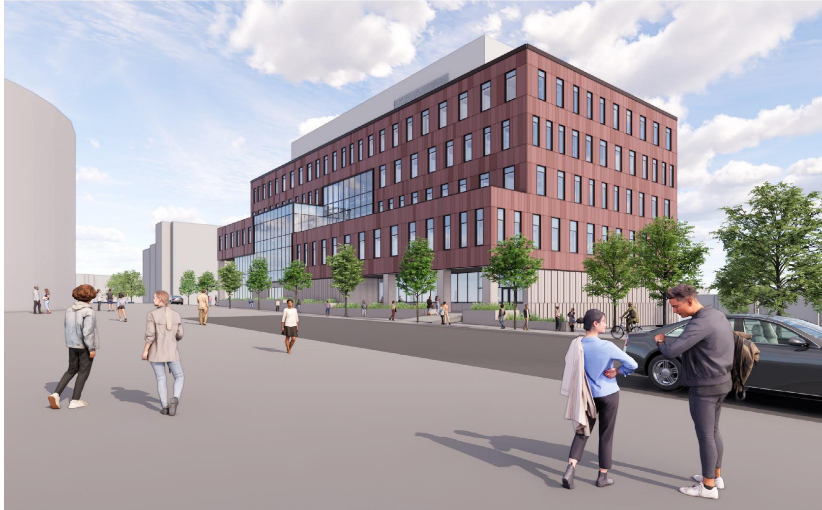
View west along W. Johnson Street
